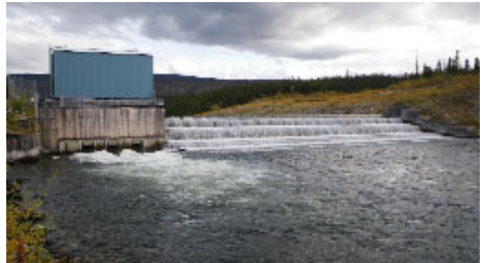
Wareham Dam. Photo: EDI Environmental Dynamics Inc.
